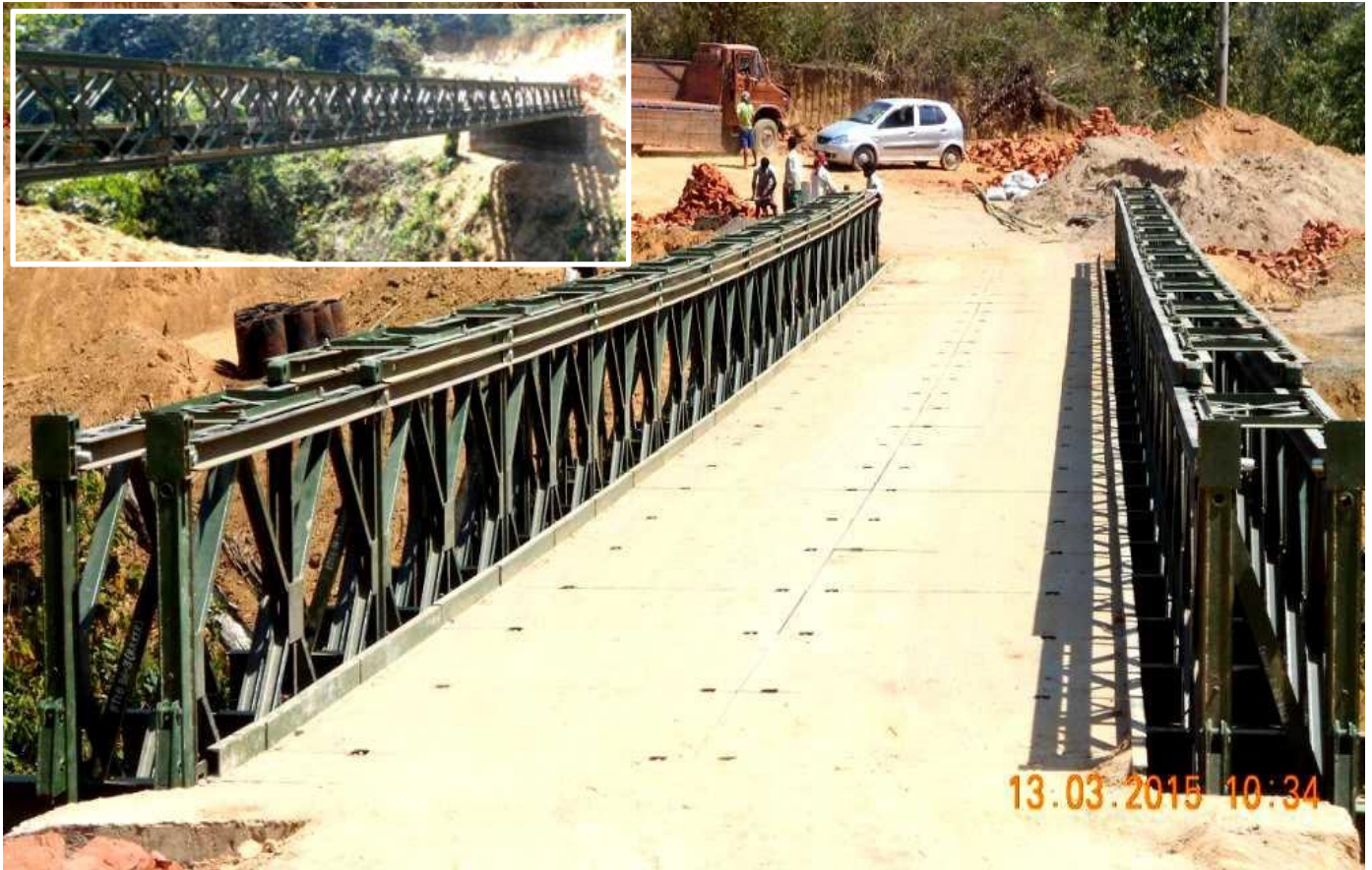
Bailey Bridge (120 ft. DSR) commissioned at Gandacherra, Tripura – for PMGSY Project
