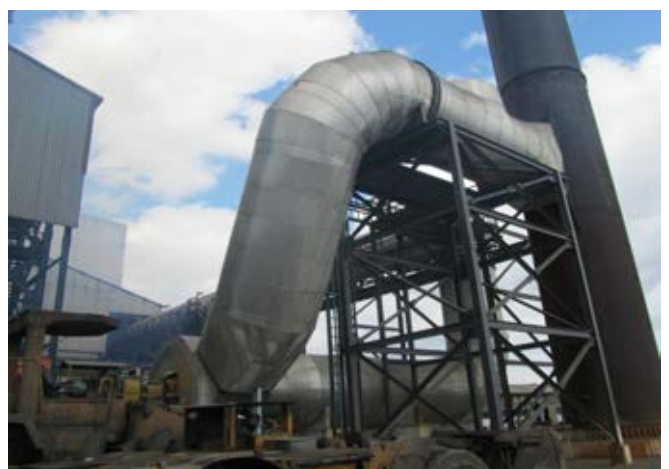
Ducts with Supporting Structure – Mopani Copper Mines, Zambia
