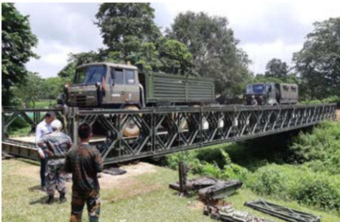
Bailey Bridge mock-erected at site by Indian Army
