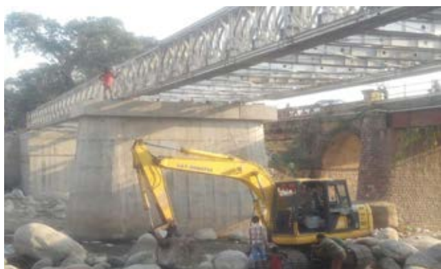
Multi-span Bailey Bridge being commissioned in Himachal Pradesh – supported by pier
